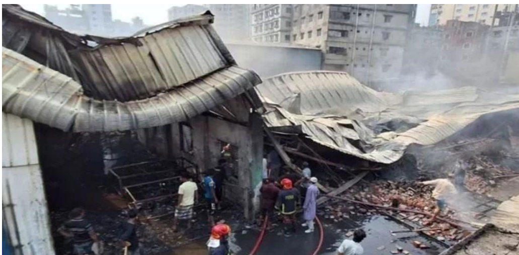
The aftermath of a fire at a gas lighter manufacturing factory in the Ambagan area of Kadamtali, South Keraniganj, Dhaka; Photo: Samakal, 5 April 2026
