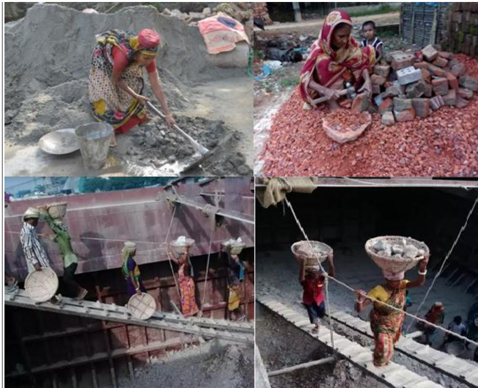
Construction workers at work (Photographs taken at Dhaka and Narayanganj).
