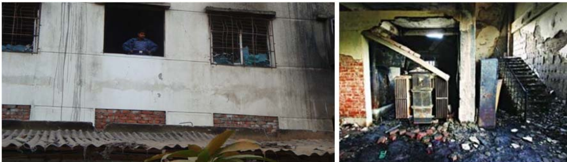
A one storied building beside the factory and another picture shows stairs of the factory (Photo: Odhikar)
