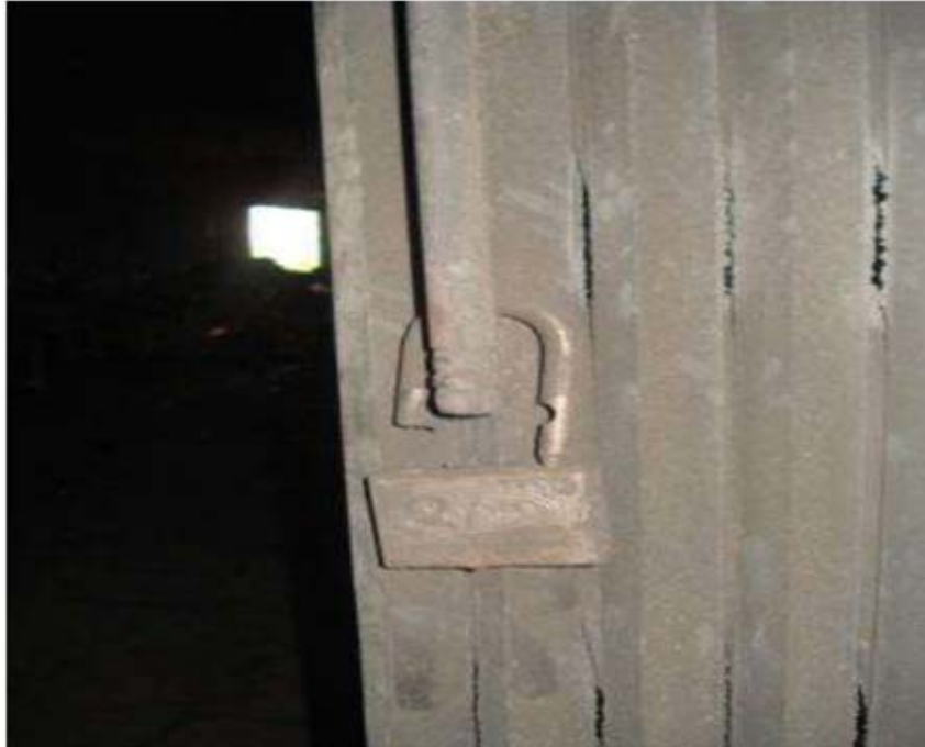
Caption: Broken padlock on the gate (Photo: Odhikar)
