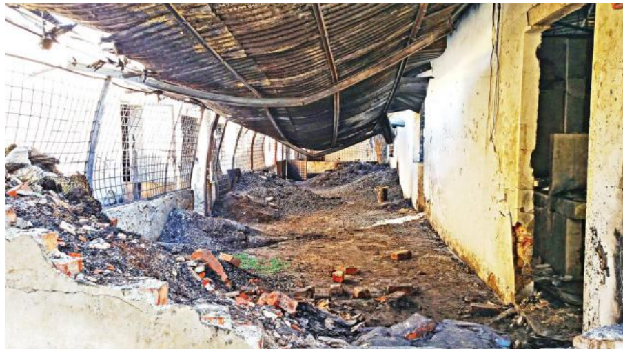
Colour match factory caught fire in Jirabo area of Ashulia, Savar, Photo: The daily Prothom Alo, 28 November 2016
