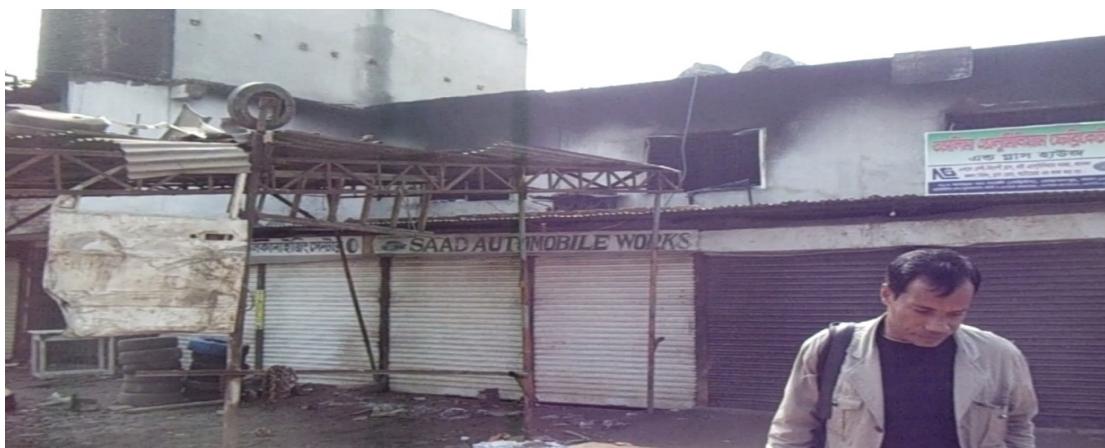
Damaged Smart Export Garments limited on the 1 st floor and automobile workshops and other shops on the ground floor (photo: Odhikar)
